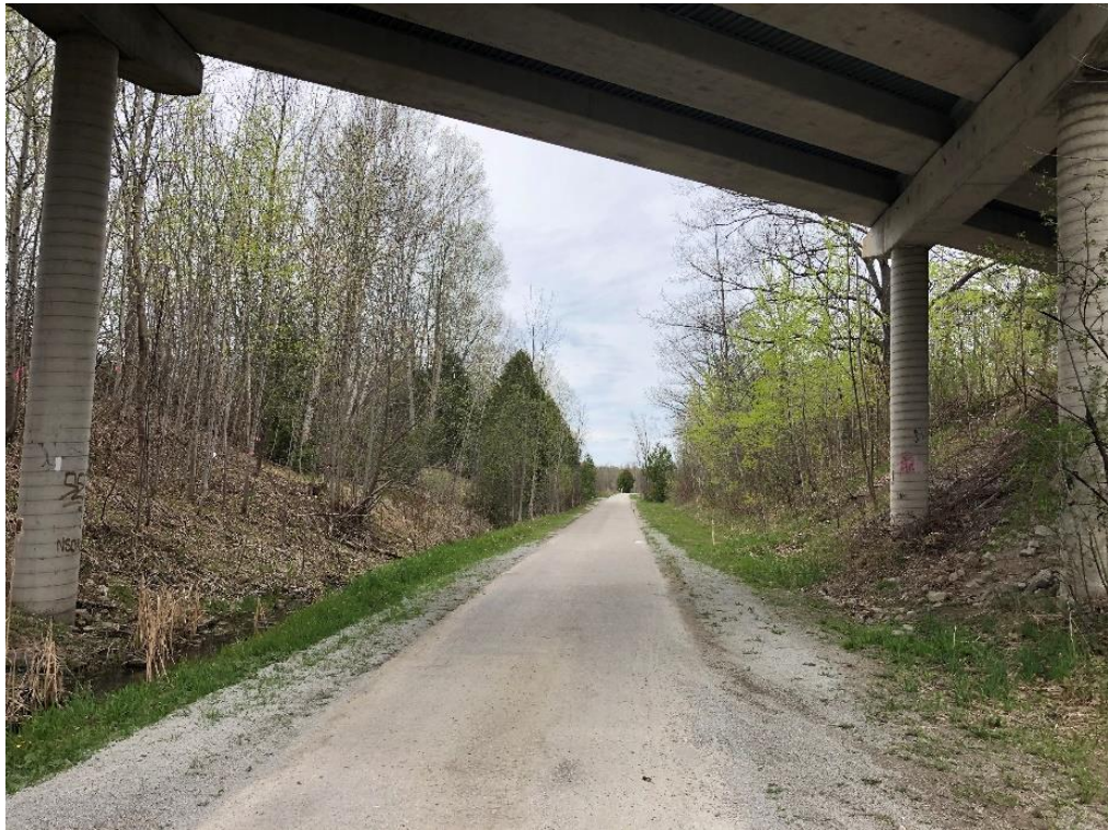
Photo 2: Photo taken from Old Fort Road Bridge facing West. March 31, 2020.
